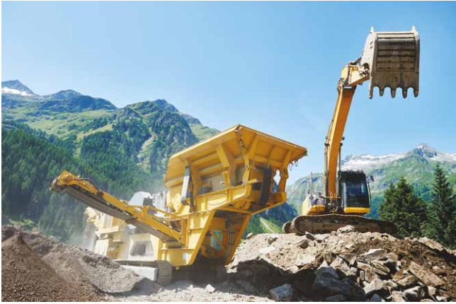
Locking a crusher flywheel using SEL4500
